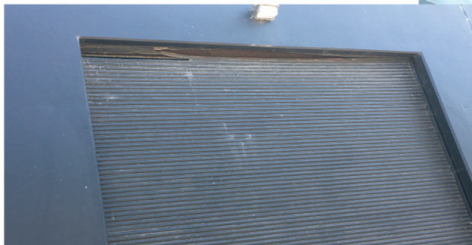
Current Project Replacing old, rusting roll-up door on north side.
